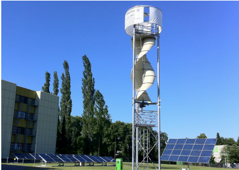
Knittelfeld - Savonius Wind Turbine and movable photovoltaic plant
